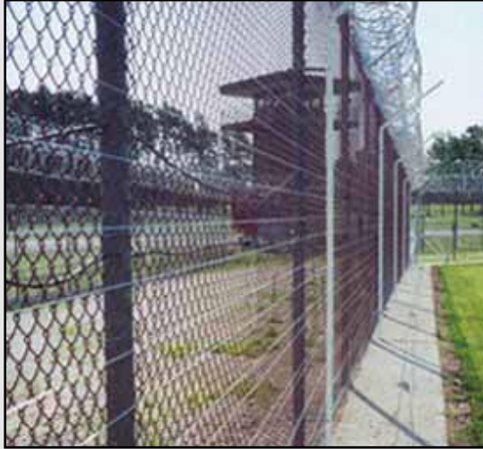
منشآت أمنية High security government facilities
